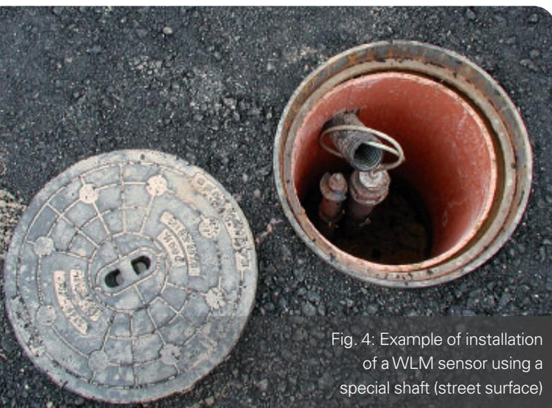
Fig. 4: Example of installation of a WLM sensor using a special shaft (street surface)
