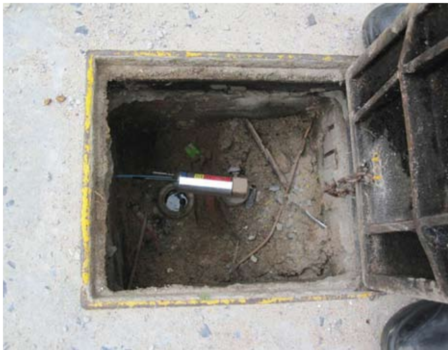
Figure 1: Logger deployment in Abu Dhabi by Gutermann
